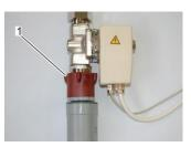
Fig. 81: Removing the safety pressure hose from the water monitor
